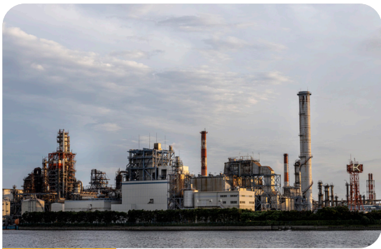
Primary & Secondary structures for boilers & turbine generators
