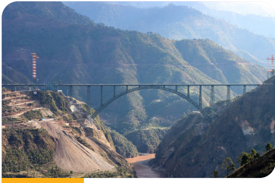
Railway bridges & girders
